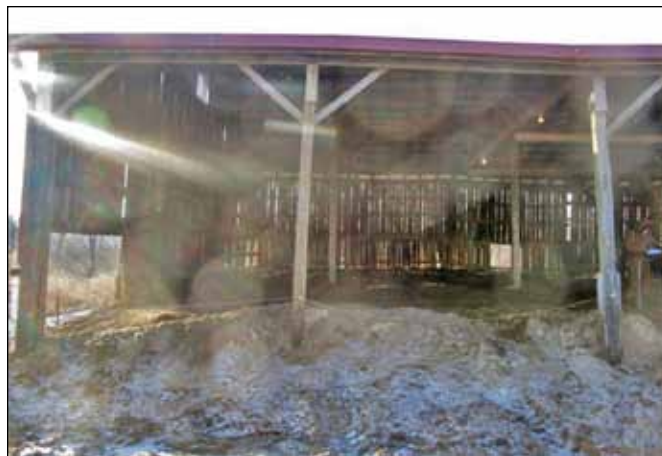
Figure 27. This barn is too closed in to allow for compost drying and air removal.
