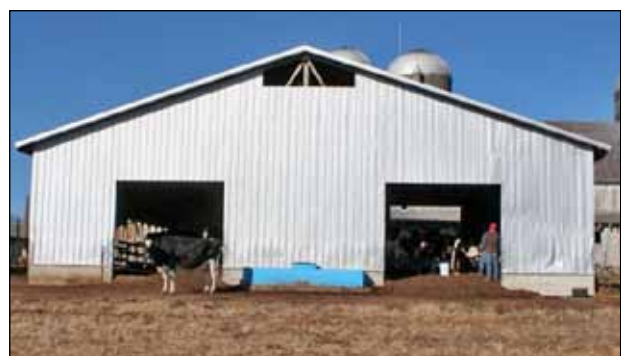
Figure 40. Each of these barns suffers from the same design flaw. In each case, the ridge opening restricts air removal from the top of the barn.
