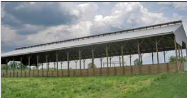
Figure 9. These facilities demonstrate features of the optimal compost bedded pack barn including high open sidewalls, open ridge with a cap, retaining walls for manure storage, and at least 100 square feet of resting space per cow.
