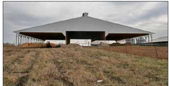
Figure 9. These facilities demonstrate features of the optimal compost bedded pack barn including high open sidewalls, open ridge with a cap, retaining walls for manure storage, and at least 100 square feet of resting space per cow.
