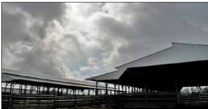
Figure 6 . These barns were constructed too close together. Neighboring barns should have at least 100 feet between them to maximize airflow.
