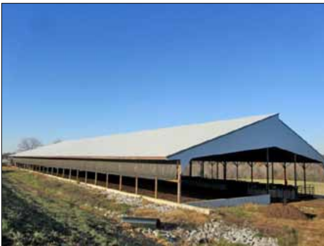
Figure 36. These designs share all the features of the first design except for the open ridge. These use an overshoot roof with an opening large enough to allow air removal from the top of the barn. The disadvantage to these is that when the wind blows toward the opening, it may actually push hot or stale air back into the barn in warmer months and cold air in the winter.
