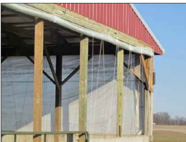
Figure 30. Cold winds blowing across the pack quickly remove the heat needed for composting. Thus, curtains are recommended in the winter. Curtains should be placed at least on the side with predominant winds.
