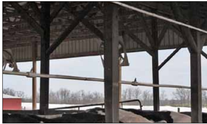
Figure 21. Sprinklers along the feedbunk, supplemented with fans, provide additional cow cooling benefits when the temperature humidity index exceeds 68.
