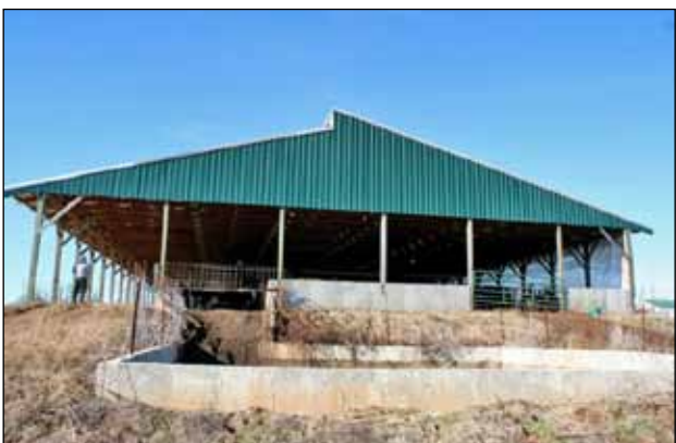
Figure 39. When the opening of the overshoot ridge is too narrow, the design restricts air removal from the top of the barn and is not generally recommend.
