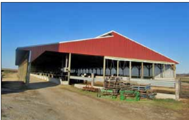
Figure 39. When the opening of the overshoot ridge is too narrow, the design restricts air removal from the top of the barn and is not generally recommend.
