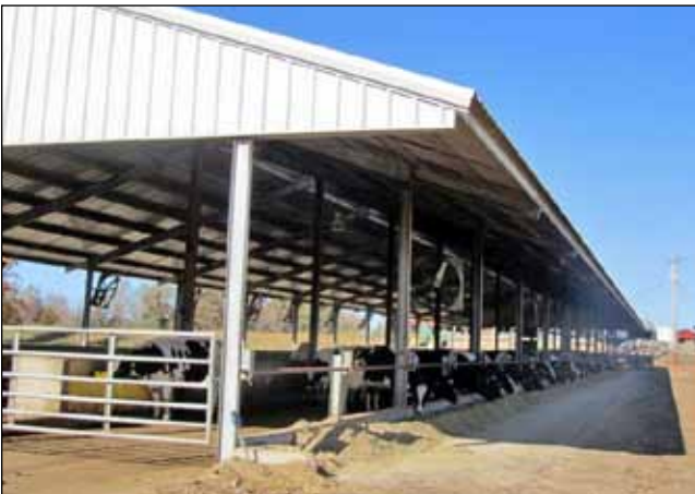
Figure 28. Eave overhangs can help minimize the amount of wind, precipitation, and sunlight entering the barn.
