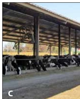
Figure 19. Drive-by or drive-through feedbunks may be used with (A) or without head locks (B and C).
