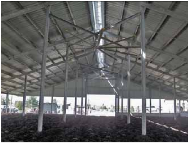
Figure 42. High volume, low speed fans have been added to many compost bedded pack barns. These fans distribute air well across a wide area.
