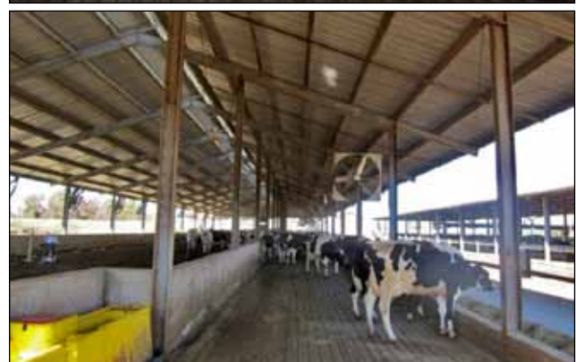
Figure 16. Wide alleys improve cow flow, minimize the risk of cow injury, and allow easy access to feed and water.
