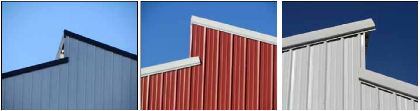
Figure 37. An overshoot roof can provide reasonable air removal when the opening is high enough as depicted in these barns. However, good air removal only occurs when wind moves across the higher side. When wind moves toward the opening, the wind actually forces air back into the barn. This design is not generally recommended.
