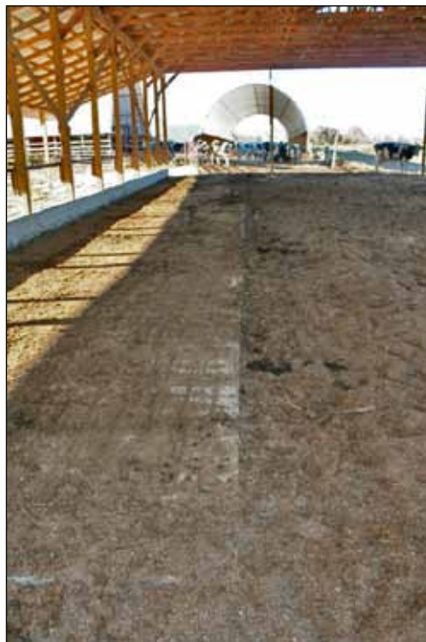
Figure 12. Without a retaining wall or fence separating the pack area from the feed alley, managing moisture in this barn may be challenging.
