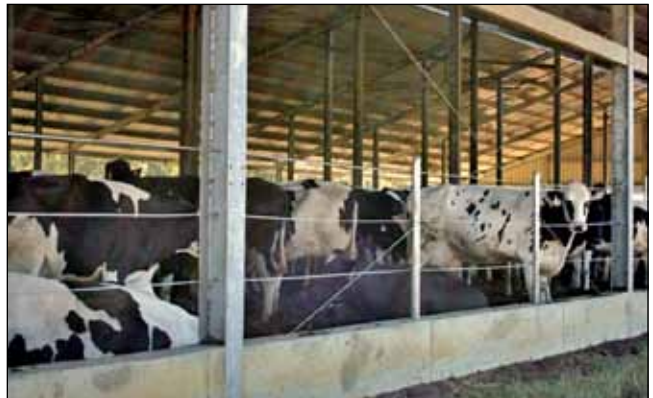
Figure 11. A concrete retaining wall provides separation between the feed alley and the pack area.
