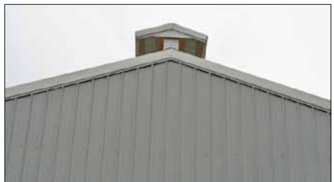
Figure 33. A ridge vent with a cap provides nearly as much air removal as the upstand with less chance of precipitation entering the barn. This design removes more air from the barn regardless of wind direction. Though this ridge vent may cost more than the overshot design, the benefits to the pack and cow performance easily outweigh the cost over the barn's lifetime.
