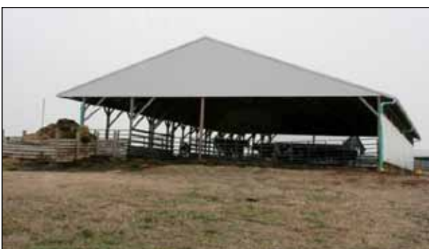
Figure 40. Each of these barns suffers from the same design flaw. In each case, the ridge opening restricts air removal from the top of the barn.
