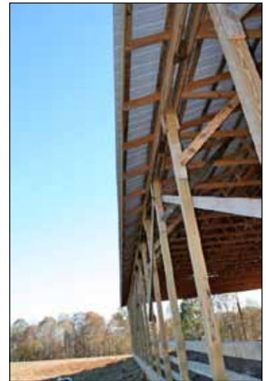
Figure 29. Short eave overhangs increase the likelihood of precipitation entering the pack and creating wet areas.
