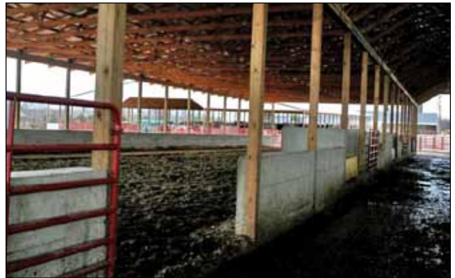
Figure 18. To minimize wetness, build multiple, narrow entrances along the long side of the barn. Entrances should be spaced every 50 feet.
