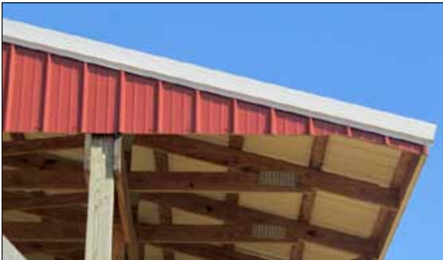
Figure 29. Short eave overhangs increase the likelihood of precipitation entering the pack and creating wet areas.
