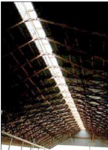
Figure 32. An open ridge vent with an upstand provides maximum air removal with minimal chance of precipitation entering the building.
