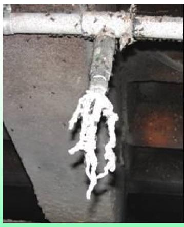
A newly installed nozzle and lateral tube next to the ESCS system (left, picture was taken on September 8), and a clogged nozzle (right, picture was taken on November 1)
